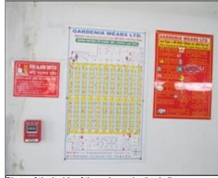
Photo of the inside of the main production hall Evacuation map.JPG
