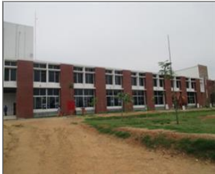
External photo(s) of the production unit(s) Building overview (2).JPG
