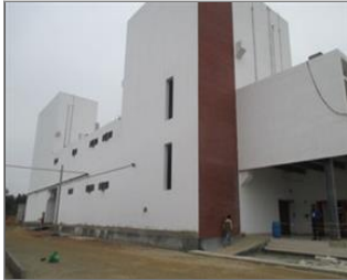
External photo(s) of the production unit(s) Back side of the building.JPG
