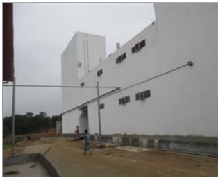
External photo(s) of the production unit(s) Building overview.JPG
