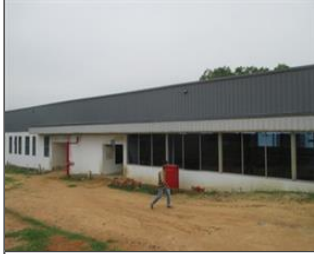
External photo(s) of the production unit(s) Facility building.JPG
